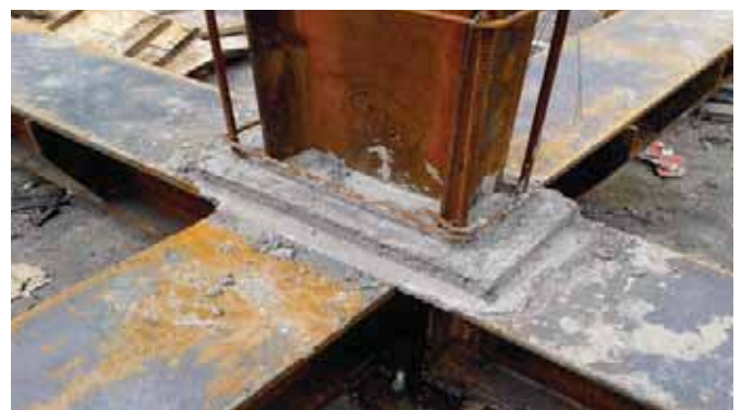
Composite column junction point
