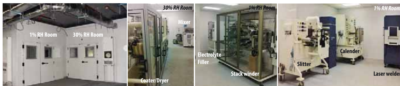
Fig. 1 Lithium-ion battery facility at CAEM, ARCI-Chennai
