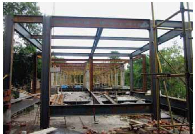
View of structural steel columns
