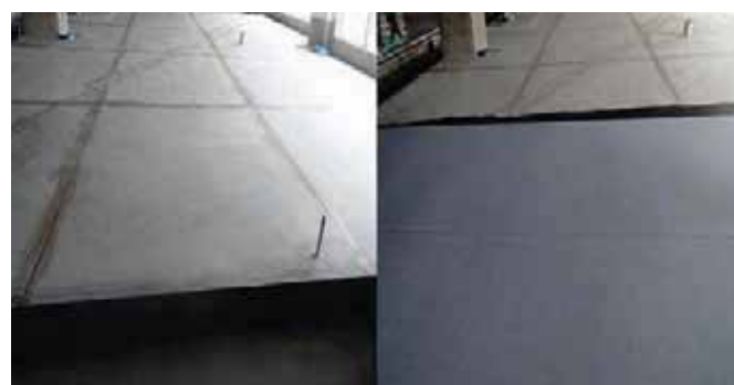
Fig. 2 Reinforced dehumidified platform laid with earthed copper sheets and electrostatic discharge mats
