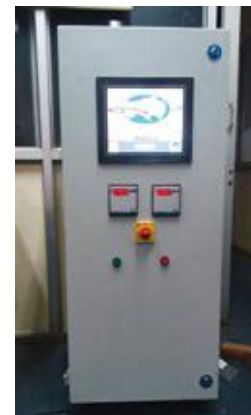
Fig.2 PLC Controlled HMI Control Panel
