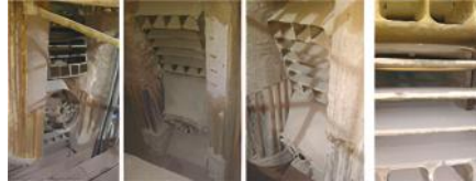
All four Burner Tips installed in Stage-I Unit-3 (Elevation-B) Boiler of 200MW NTPC-Farakka Thermal Power Plant
