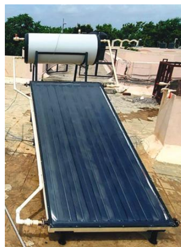
\text{CuMnNiO}_4 Spinel nanoparticles based absorber coated Flat plate collector
