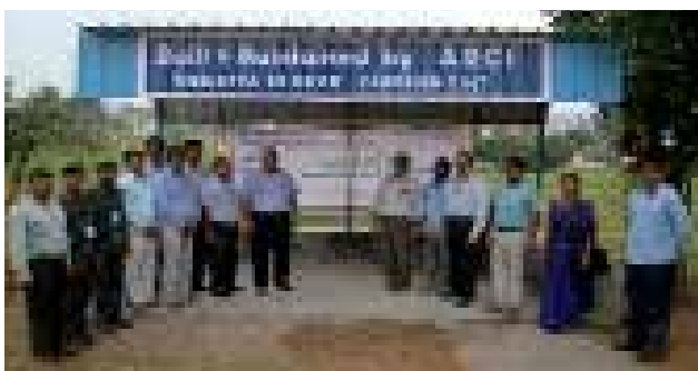
Renovated bus shelter opposite ARCI premises
