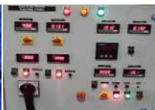
Exclusively designed and custom built 30 kVA MAO control system
