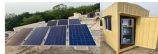
PV-Performance monitoring system for validation of PV Panels
