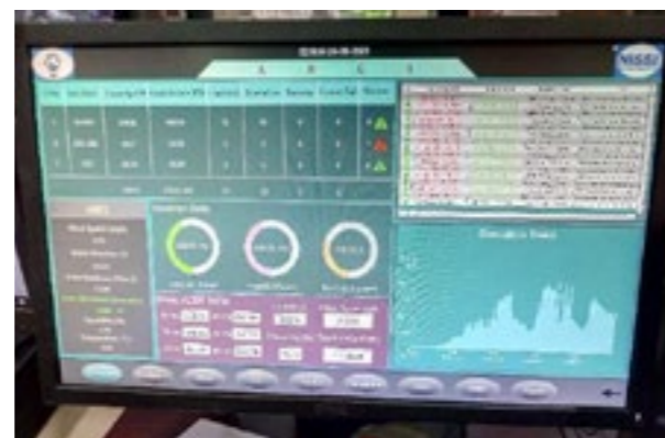
SCADA user interface of 518 KWp solar plant
