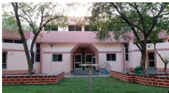
Refurbished canteen building
