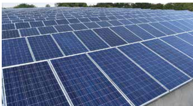
Solar roof top power plant
