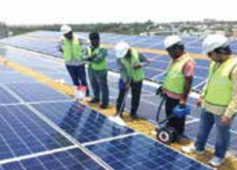
Coating demonstration on roof top of PV power plant
