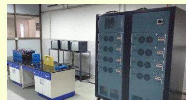
LIB pack testing facility
